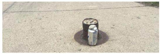
A metal pipe filled with cement protrudes from the center of a sidewalk panel. An ordinary 12-ounce soda can is placed next to the pipe for scale, showing that the pipe is slightly taller and about twice as wide as the can.
