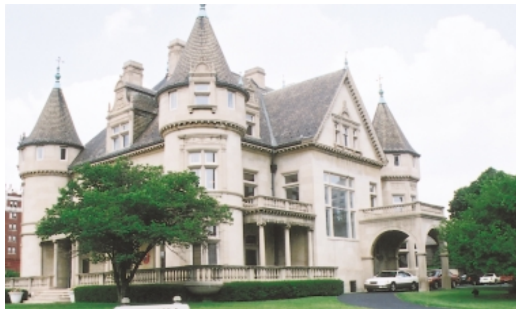
The Hecker-Smiley mansion has an Indiana limestone exterior and gray slate roof. Round corner towers, filials, and other ornate features give the building its grand appearance.
