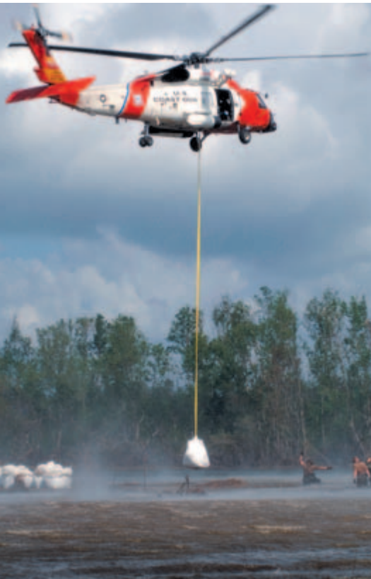
Coast Guard helicopter assists in the repair of the New Orleans levy break.
