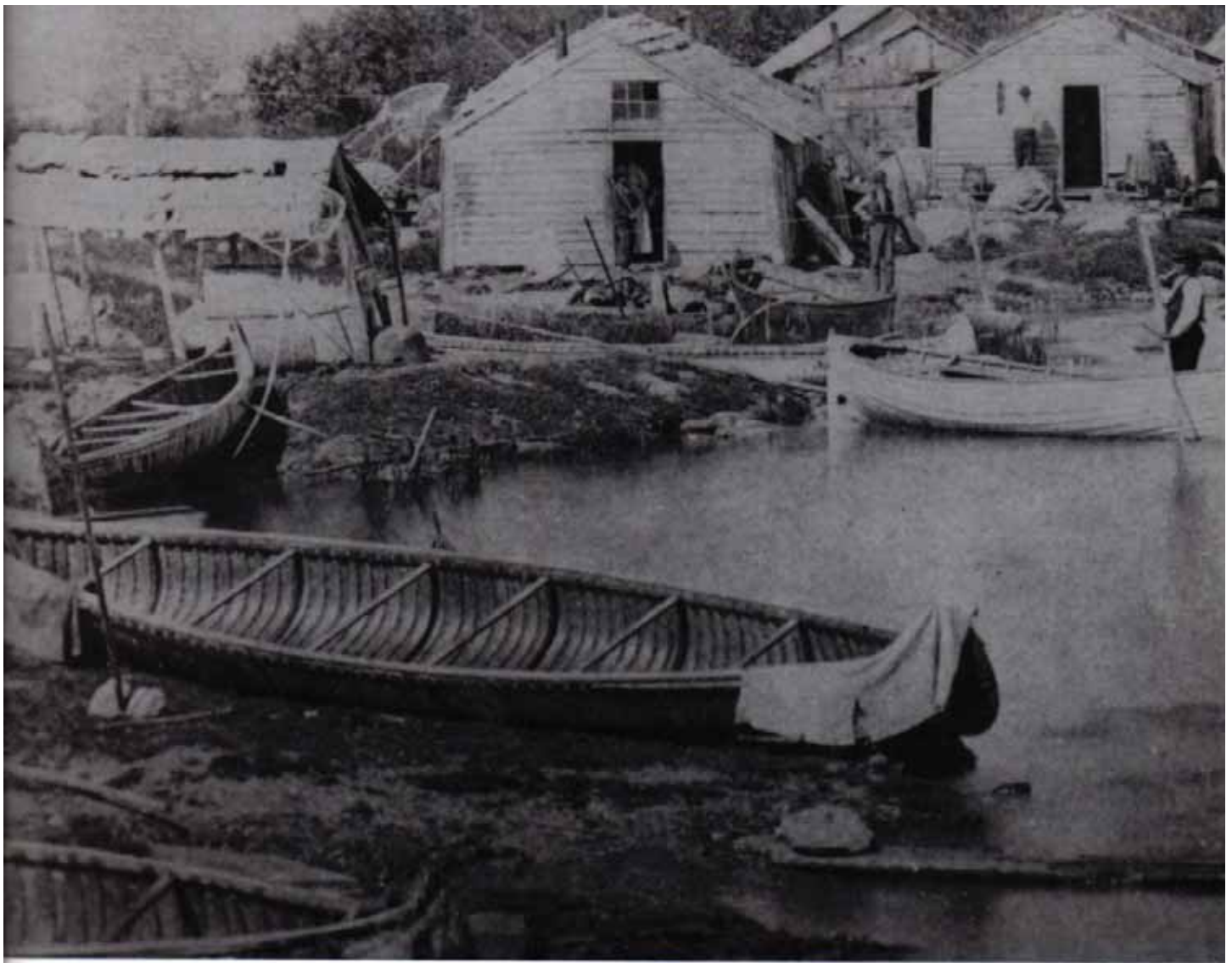
Pond's demolished net house (upper left) and home (to its right) can be seen in this photo of the fishing village at Seul Choix. Courtesy of Jerry Pond.
